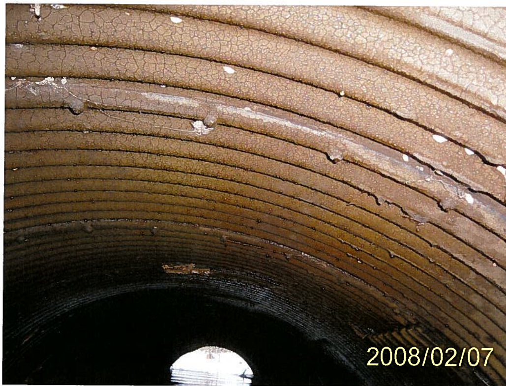
Photo 6: Structure C01 – Culvert barrel interior.
