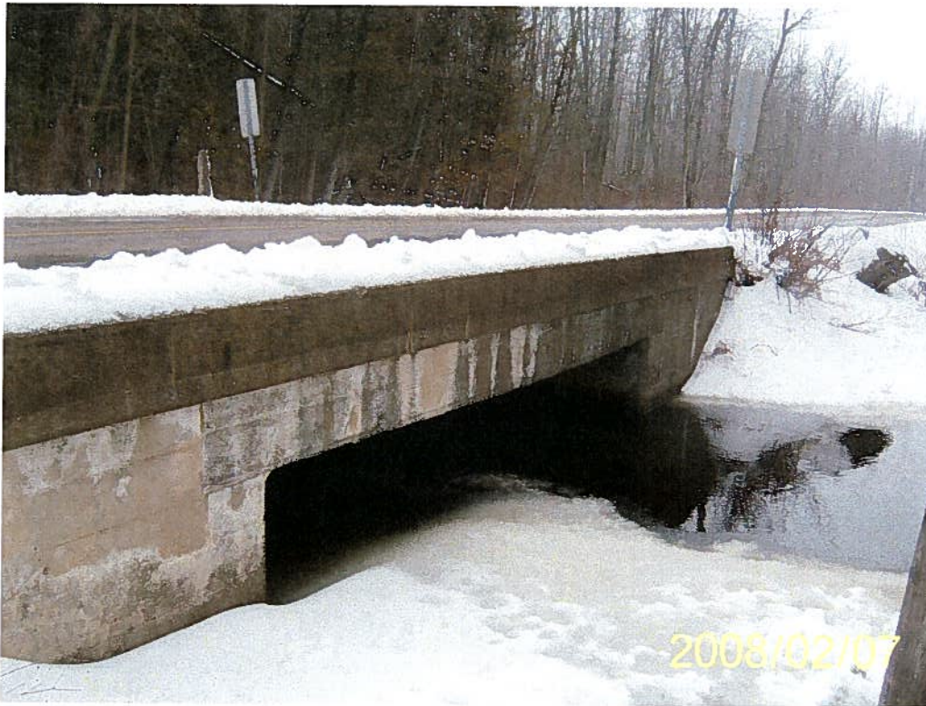
Photo 12: Structure C03 – Elevation.
