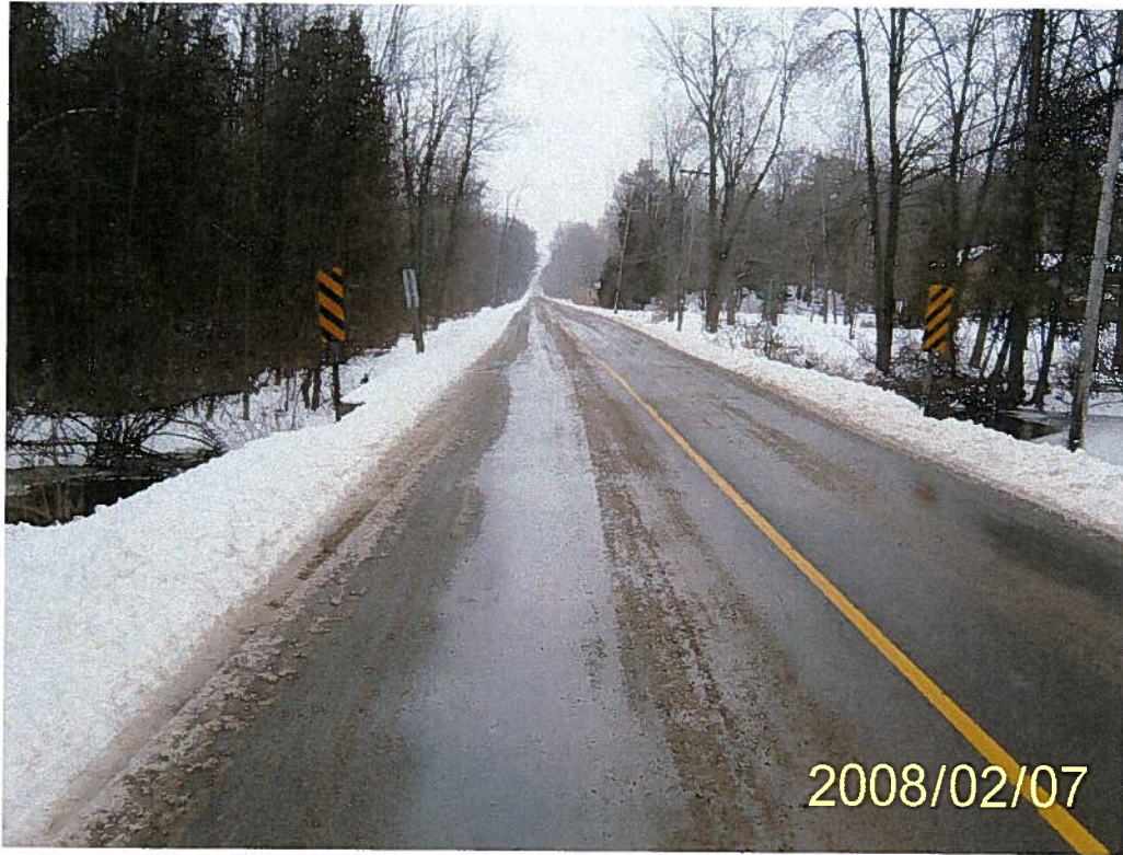
Photo 11: Structure C03 – View of road over structure.
