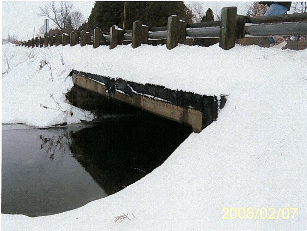
Photo 15: Structure C04 – Elevation.
