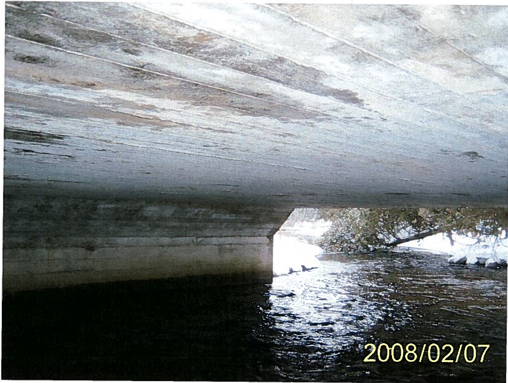
Photo 9: Structure C02 – Structure interior.
