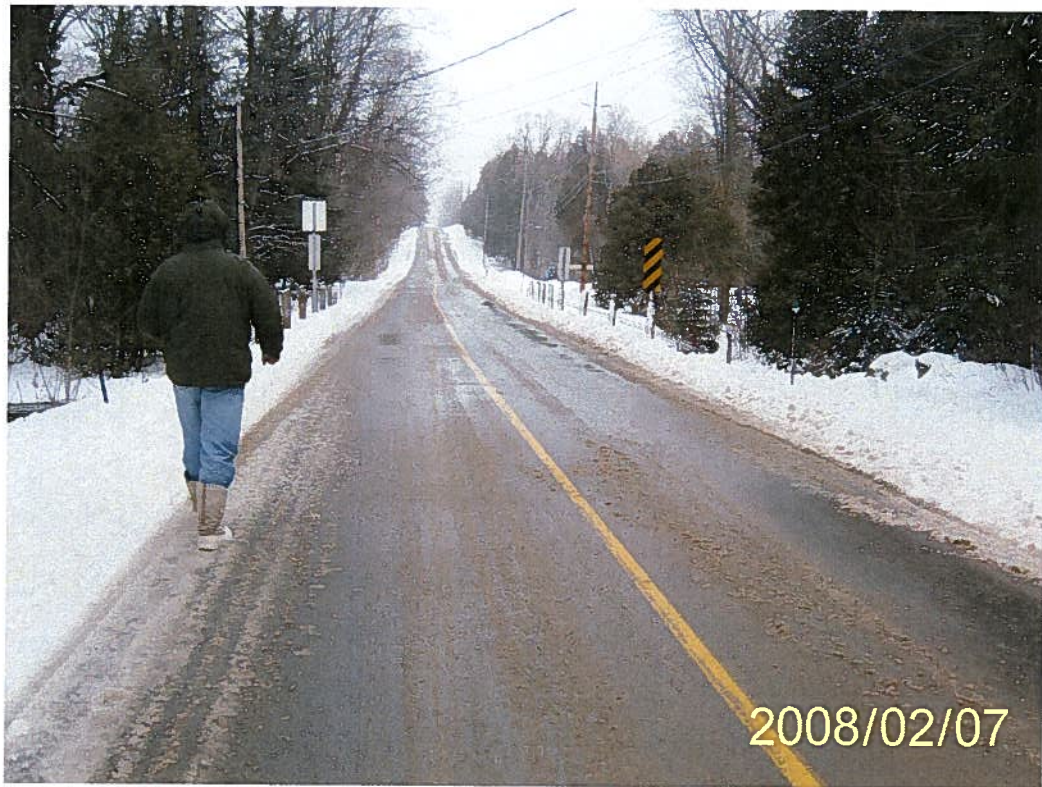
Photo 7: Structure C02 – View of road over structure.
