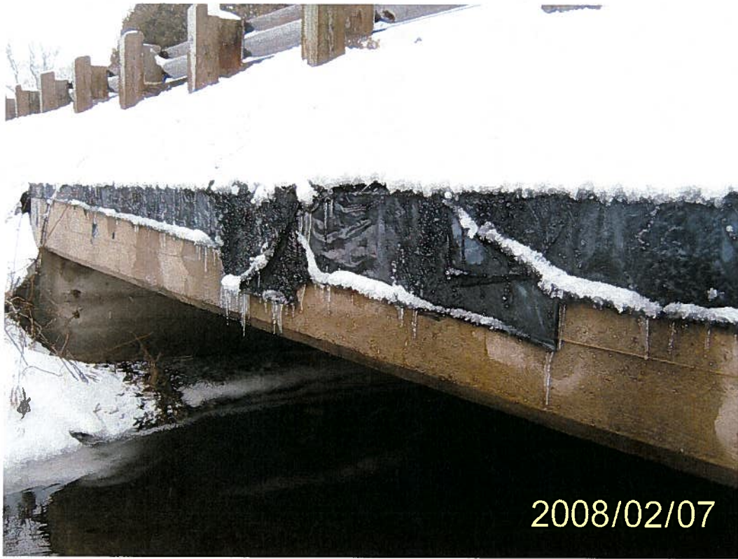
Photo 17: Structure C04 – Structure fascia.
