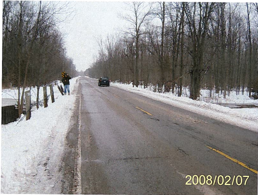
Photo 1: Structure C01 – View of road over structure.
