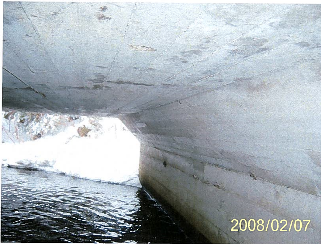
Photo 10: Structure C02 – Structure interior.
