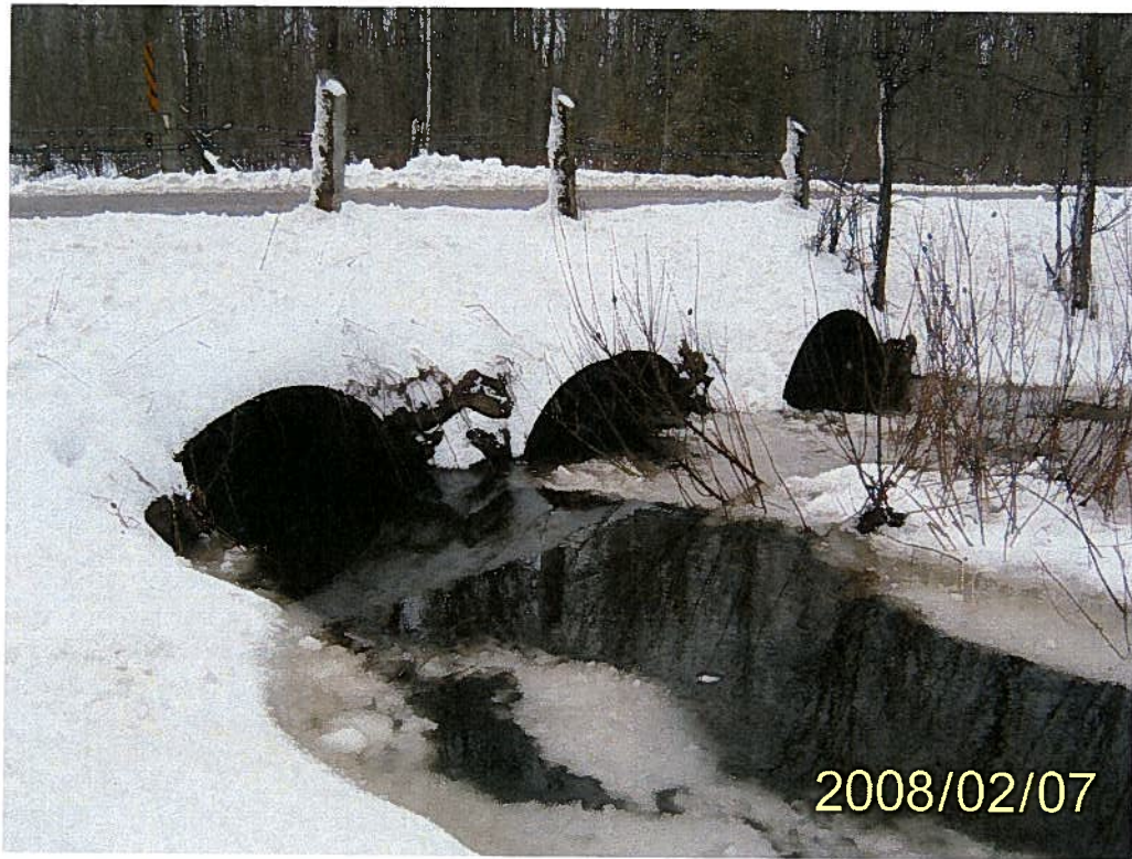
Photo 2: Structure C01 – Elevation.
