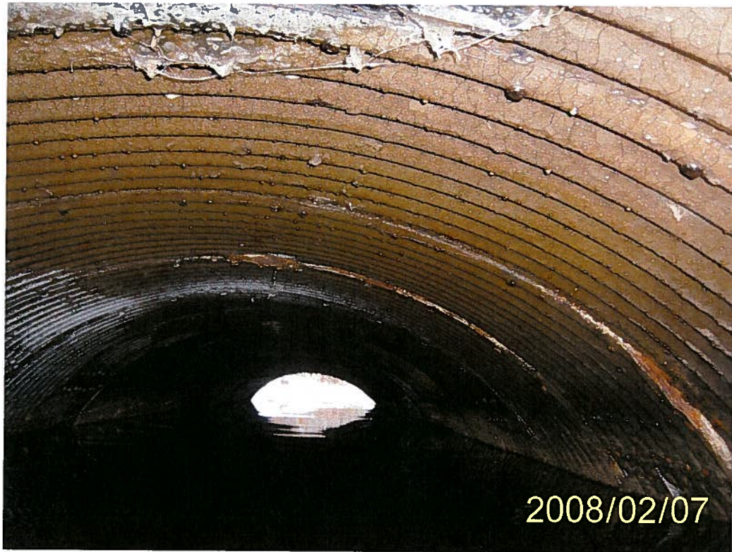
Photo 3: Structure C01 – Culvert barrel interior.
