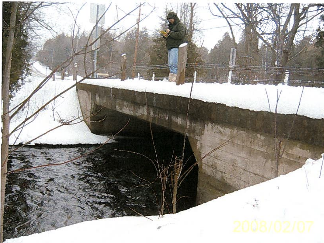
Photo 8: Structure C02 – Elevation.
