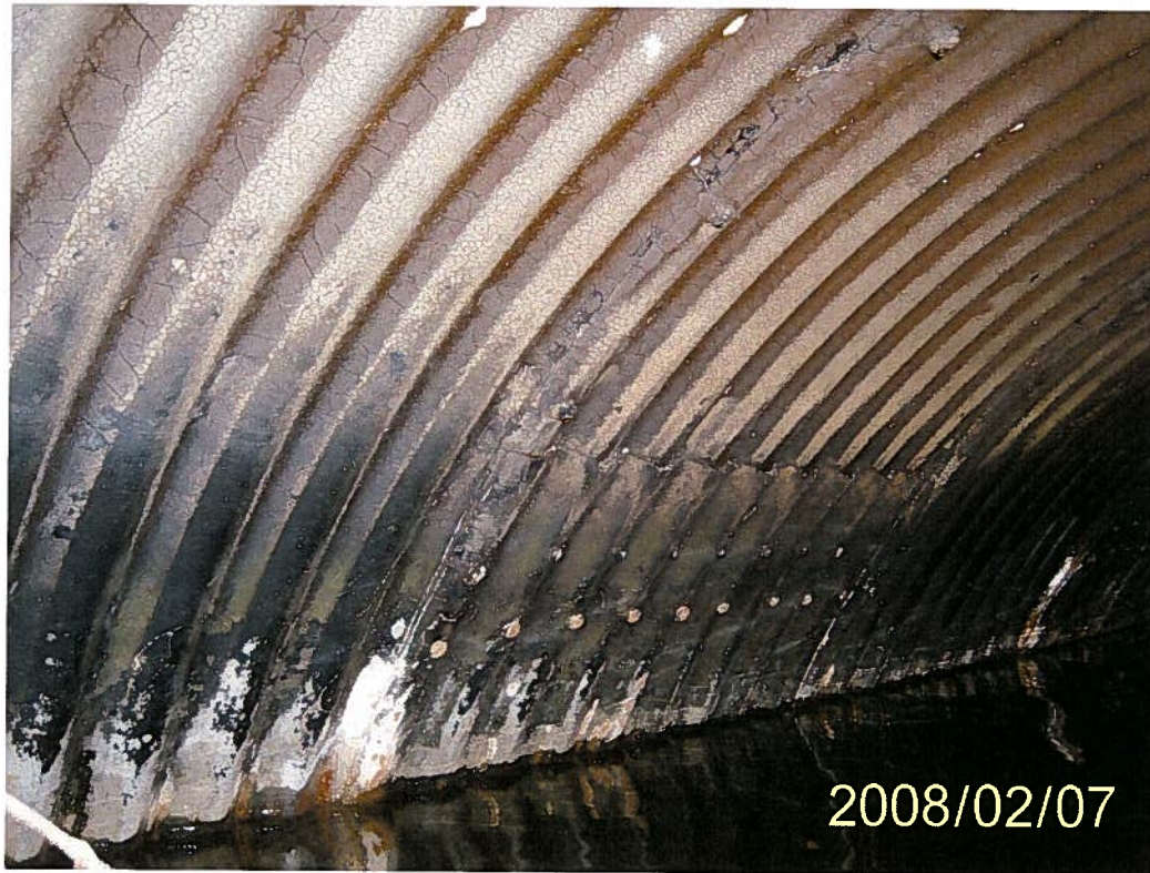
Photo 5: Structure C01 – Culvert barrel interior.
