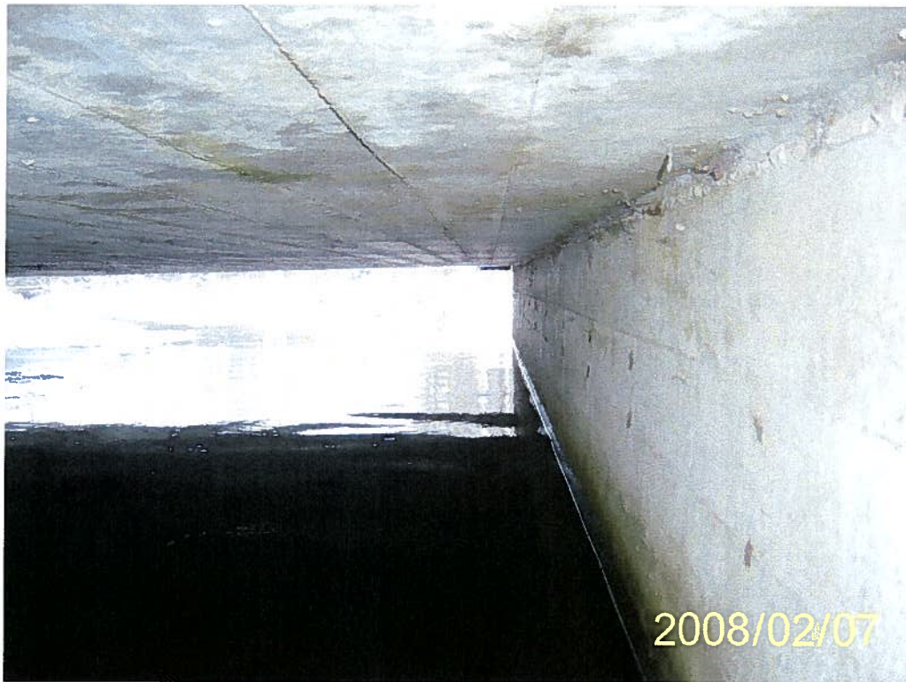
Photo 16: Structure C04 – Structure interior.
